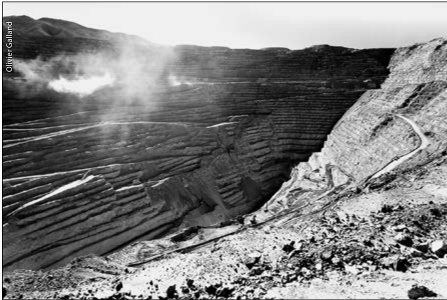
The Chuquicamata copper mine, a 4.3-km long, 3-km wide and 1-km deep hole. In the shaded part of the mine, between the white dust cloud and the right flank, a darker steeply-dipping track, ending up in collapse deposits near the bottom of the mine, is visible: it is the trace of the fault that controlled the emplacement of the magmatic intrusions and the ore.
