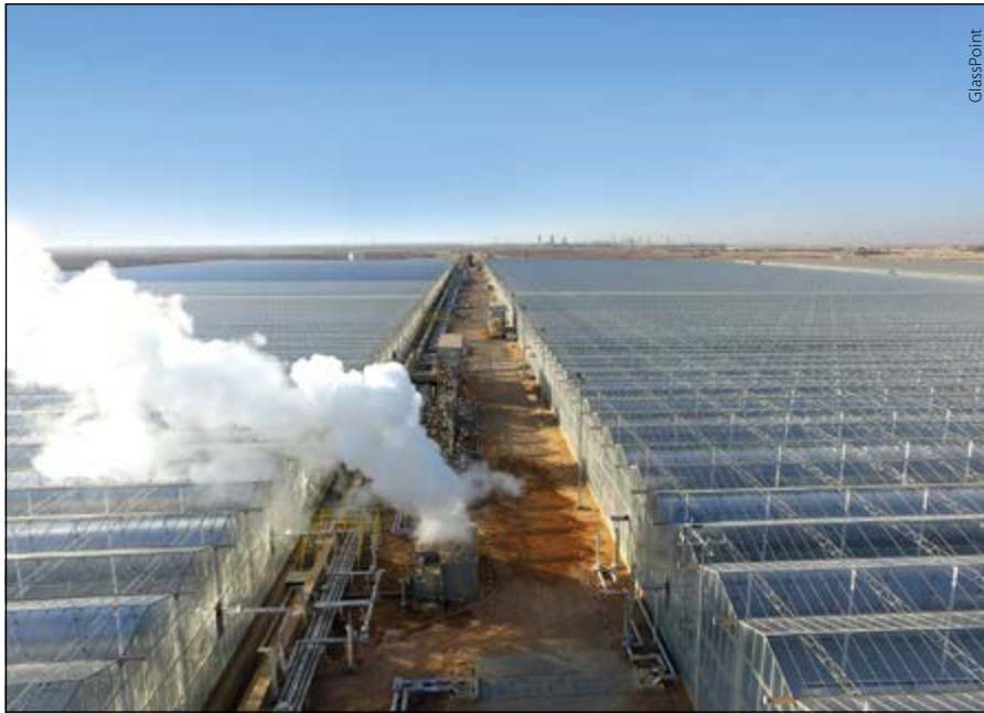
Huge greenhouses protect the steam-generating mirrors in the Miraah project.
