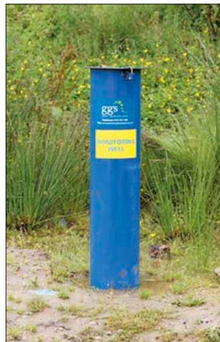
Unobtrusive borehole monitoring
