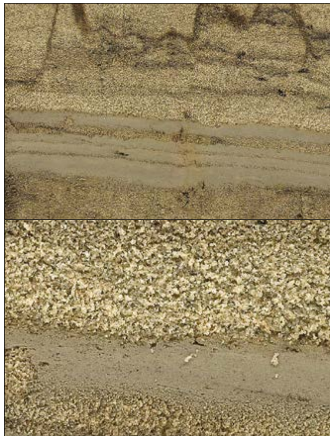
Standard 300 dpi 'high-resolution' imagery (top) compared to the 1,360 dpi resolution available using the TenEx imagery system (bottom).
