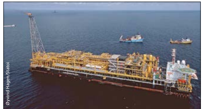
The Girassol FPSO
