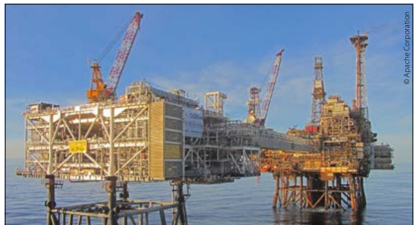
The new Forties Alpha Satellite Platform bridge linked to the Forties Alpha platform.
