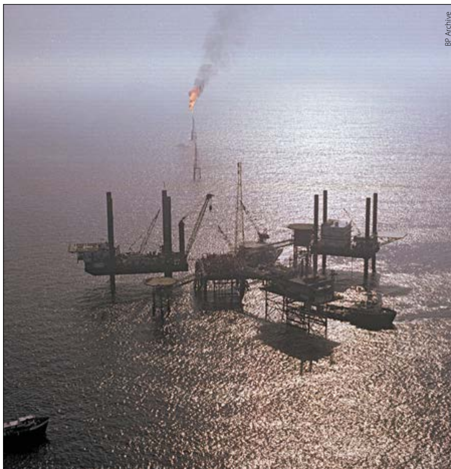
The Zakum Central Supercomplex in 1979.
