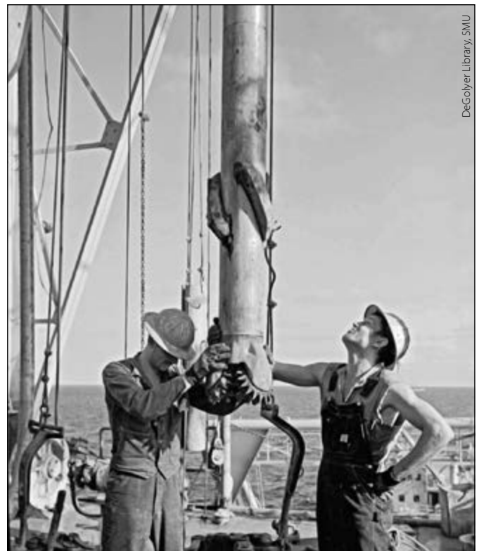
Workers guiding the bottom hole assembly with stabilizer and new rock drill bit on an offshore drilling platform, 1955.
