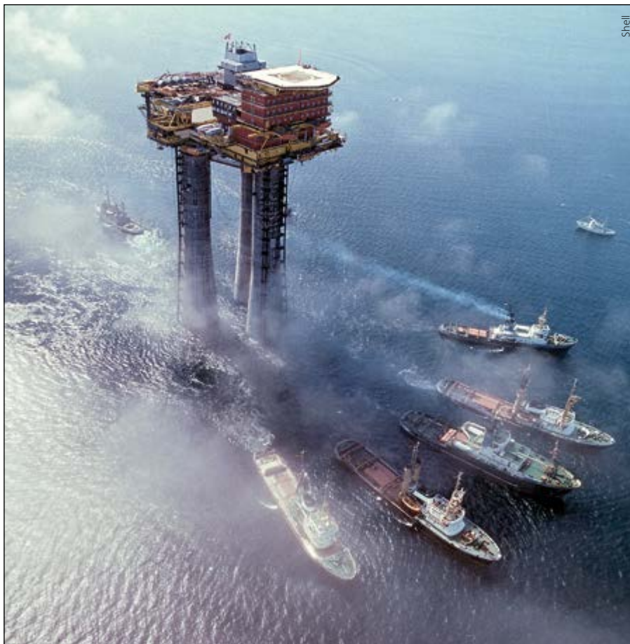
Brent B, the first Brent platform to be commissioned, was built in Stavanger, Norway and towed out to its location on the field in August 1975.
