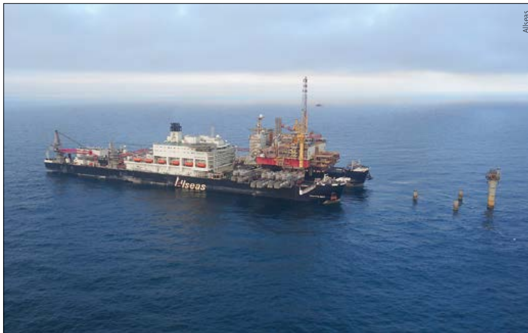
The specially built decommissioning vessel Allseas 'Pioneering Spirit' can remove the topsides of a platform in a single lift. Here it is seen carrying the structure of the Norwegian Yme field platform.
