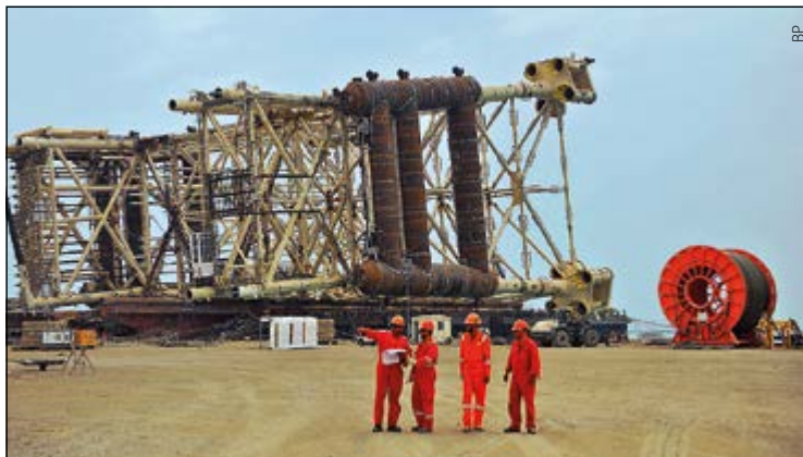
The first Shah Deniz 2 platform before it was transported out to the field.
