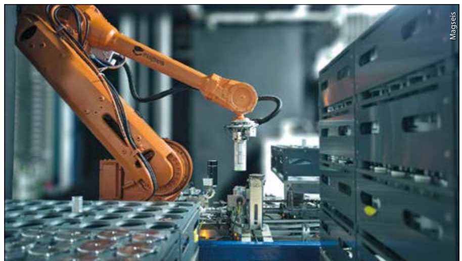
One of the docking robots onboard handling control units and battery units.
