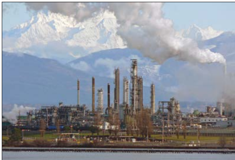
The Anacortes refinery in Washington state, where seven workers died in 2010 when a heat exchanger violently ruptured after a maintenance restart.
