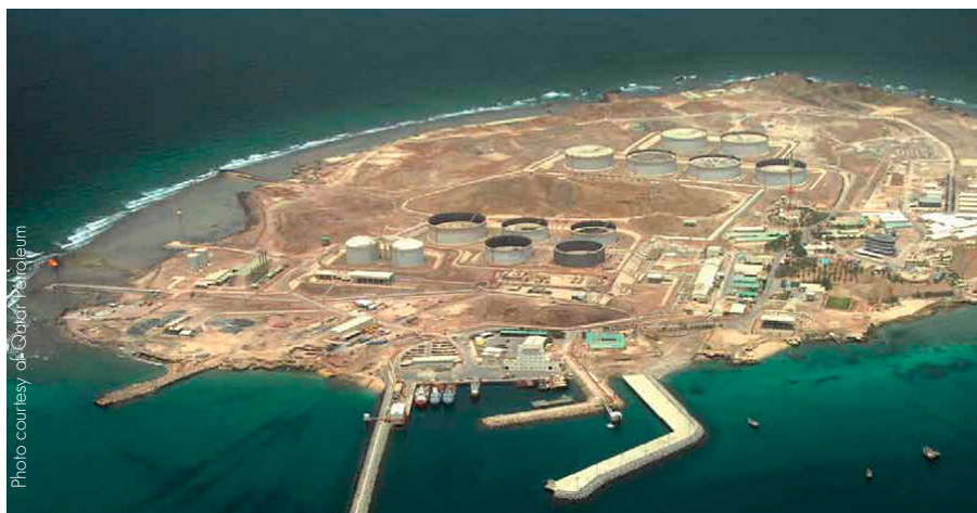
A view of Halul Island (an area of 1.5 sq. km) from where the first shipment of oil produced by Shell from the Idd al-Sharqi field was exported on 1 February 1964. Today, the island is home to 11 large oil storage tanks with a total capacity of 5 million barrels; it also has pumping stations and modern loading terminals for tankers. In 2008, oil exported from Halul was about 90 million barrels transported by 137 tankers; operations are managed by the Qatar Marine Crude.
