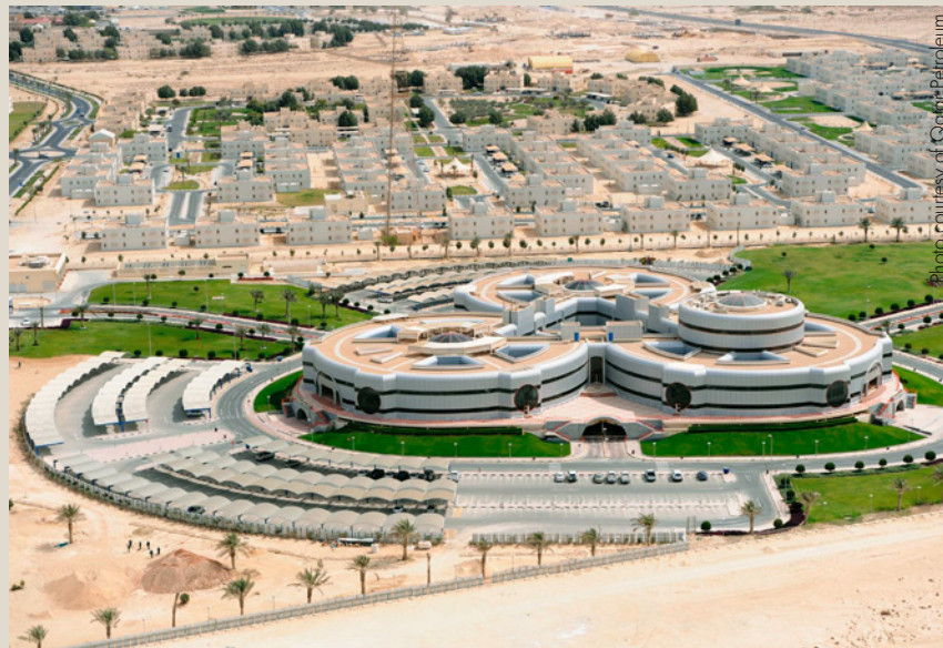
A view of the new Qatar Petroleum corporate training facility at Dukhan
