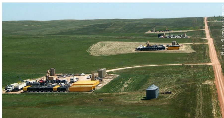
A simultaneous frac of three wells in the Bakken Formation in Montana. The wells are separated by 400 m and the horizontal bores are perpendicular to the section line road. The length of the view down the road to the horizon is roughly half the distance traversed by the horizontal well bores. The 2,700 m distance more than doubles the lateral lengths of the early wells. Stimulation size has increased as well, from 136 metric tons of sand to as high as 635 metric tons.
