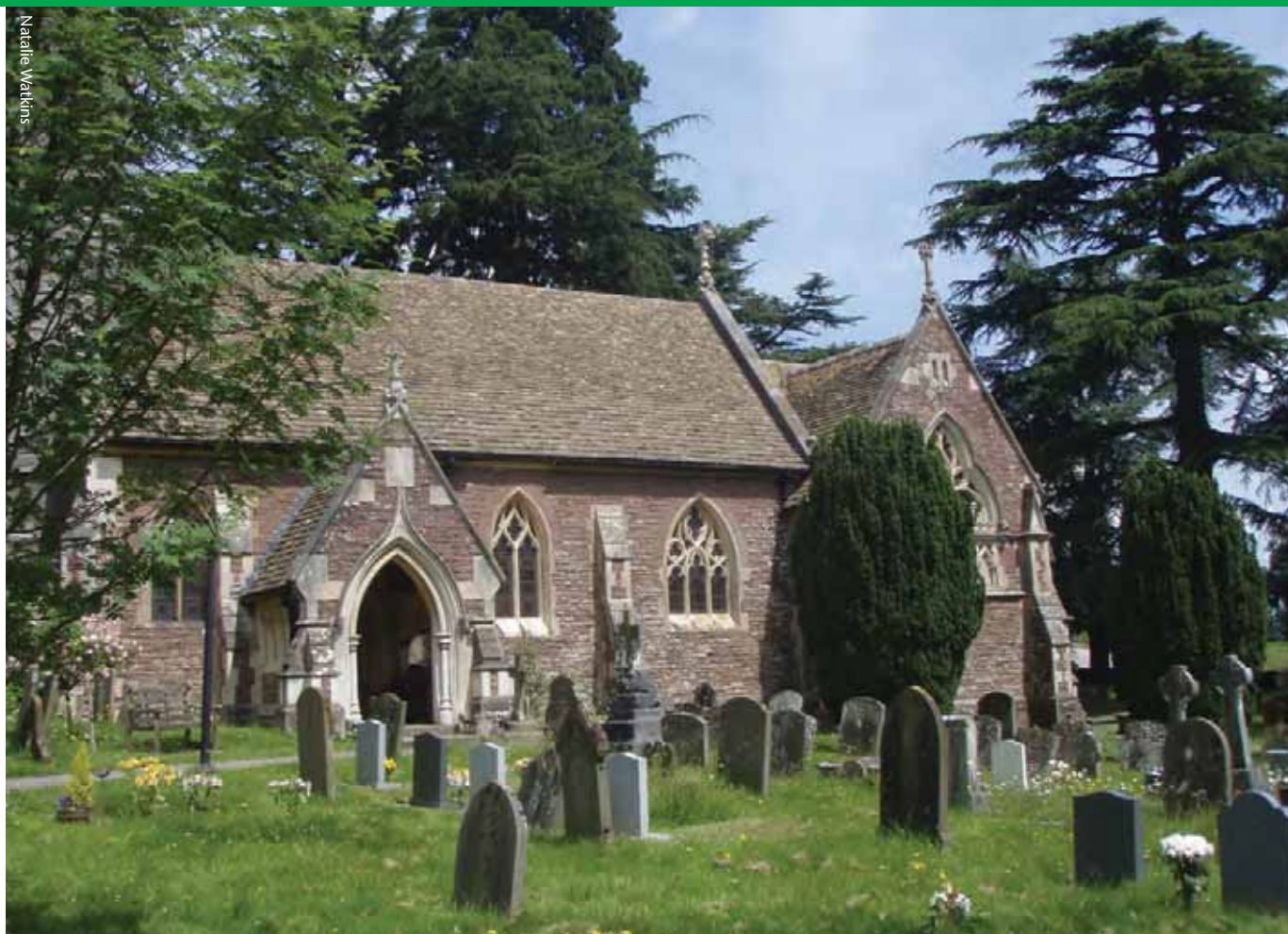
Huntley church, near the southern end of the trail, is built from the wonderful combination of Triassic red sandstone and Jurassic limestone.
