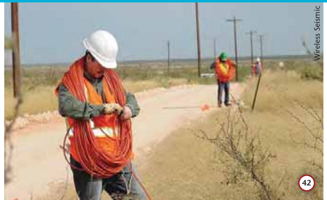
'Juggies' laying cables for a land geophysical survey – but is the age of seismic upon us?
