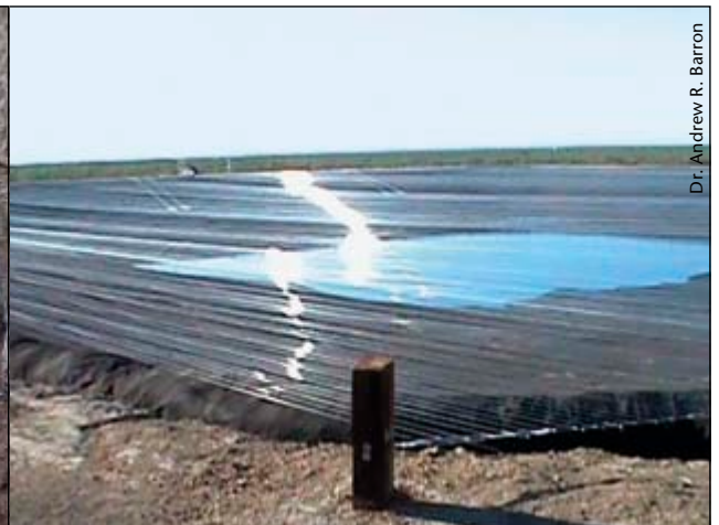
Fracture fluids are often sprayed into visqueen-lined pits (left) that can leak. The poly-asphalt containment pit (right) may cost twice that of visqueen-lined pits but provides a containment system very resistant to wear and corrosion. This pit has a grid added above it to protect wildlife.
