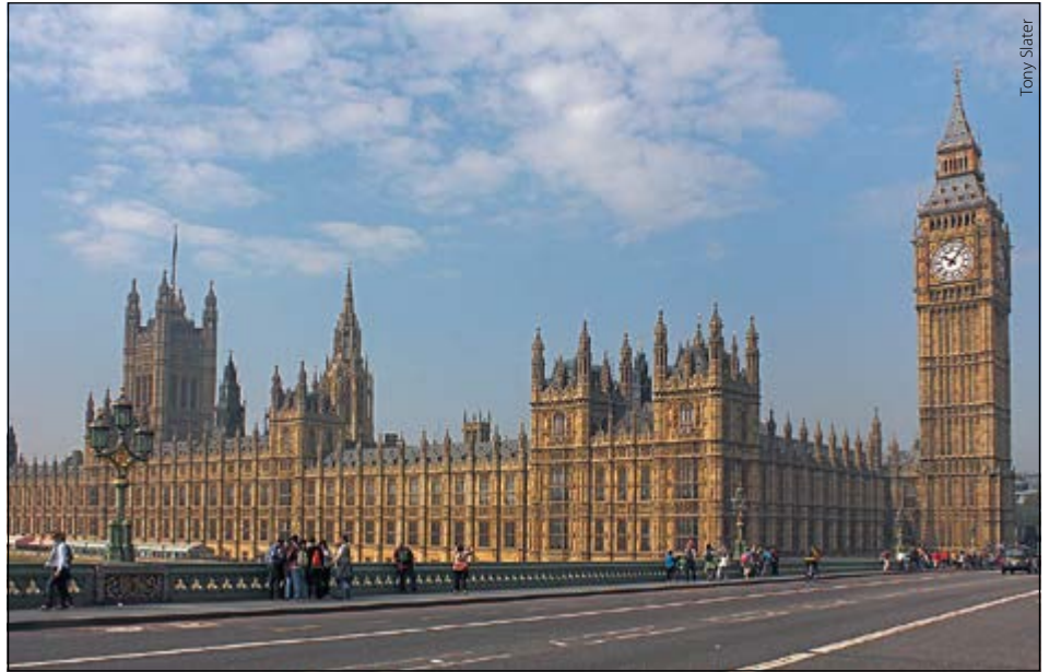
The Houses of Parliament: Permian Anston Limestone from a quarry in South Yorkshire.
