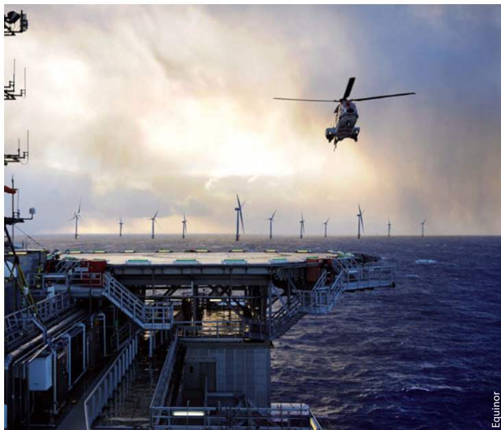
Hywind Tampen is an 88 MW floating wind power project intended to provide electricity for the Snorre and Gullfaks offshore field operations in the Norwegian North Sea. It will be the world's first floating wind farm to power offshore oil and gas platforms.
