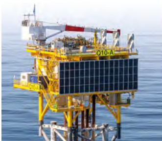
Figure 2: Block Q10-A unmanned platform with solar panels and wind turbines.
