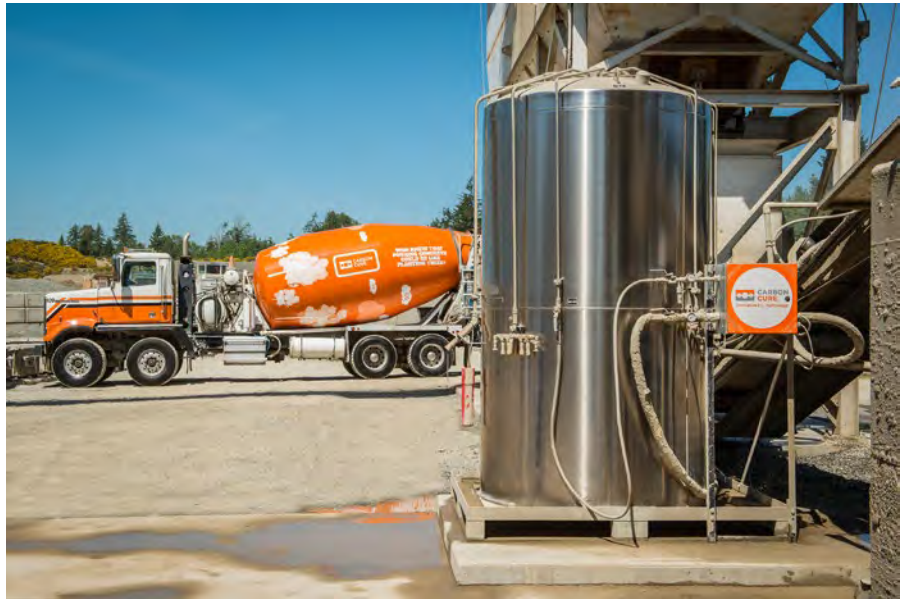
| A CarbonCure truck carrying CO 2 -cured concrete.
