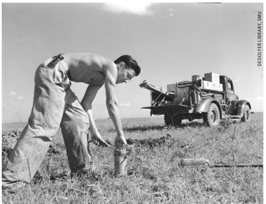
| A worker placing explosives for seismic testing, 1940.
