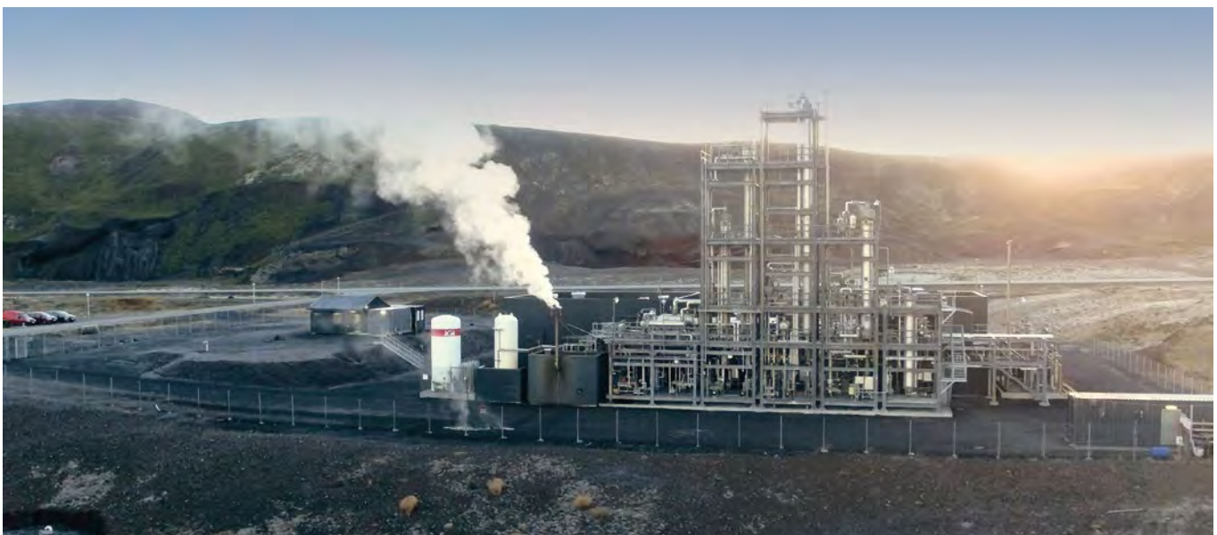
| The George Olah plant in Iceland creates methanol from geothermal power plant emissions.
