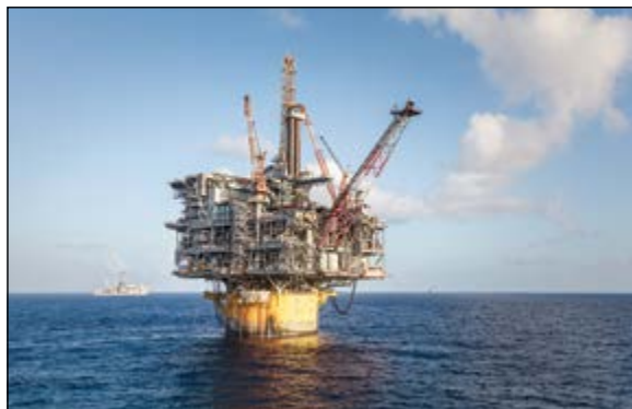
In 2,450m of water, Shell's Perdido is the world's deepest spar, and the second-deepest oil and gas production hub.
