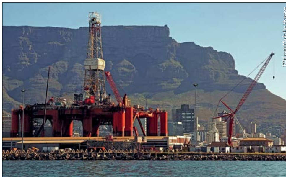
Rig being repaired in the port at Cape Town, South Africa.
