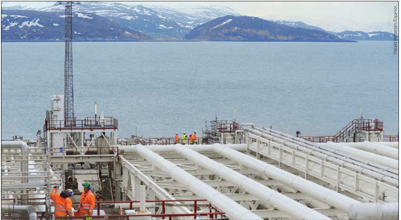
Gas is piped from the Barents Sea Snøhvit field to the Melkøya LNG processing plant, where the CO 2 is separated out and sent back to be injected into the depleted reservoirs.
