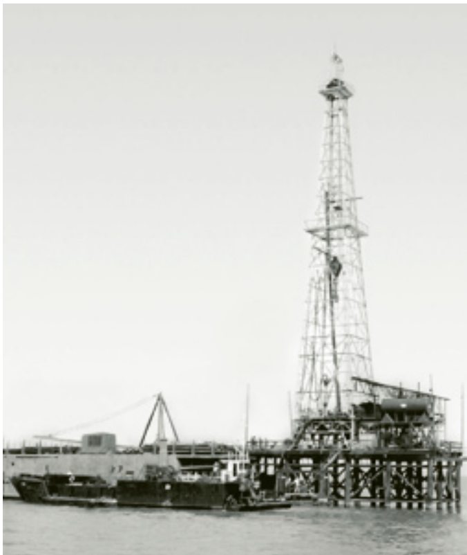
The historic first offshore discovery out of sight of land was completed in 1947 by Kerr McGee Rig 16, a new concept using a mobile drilling 'tender'. Off southeast Louisiana, the Ship Shoal 32 well was drilled to a total depth of 770 m in 4 m of water 14 km from shore. The field produced oil until 1984.
